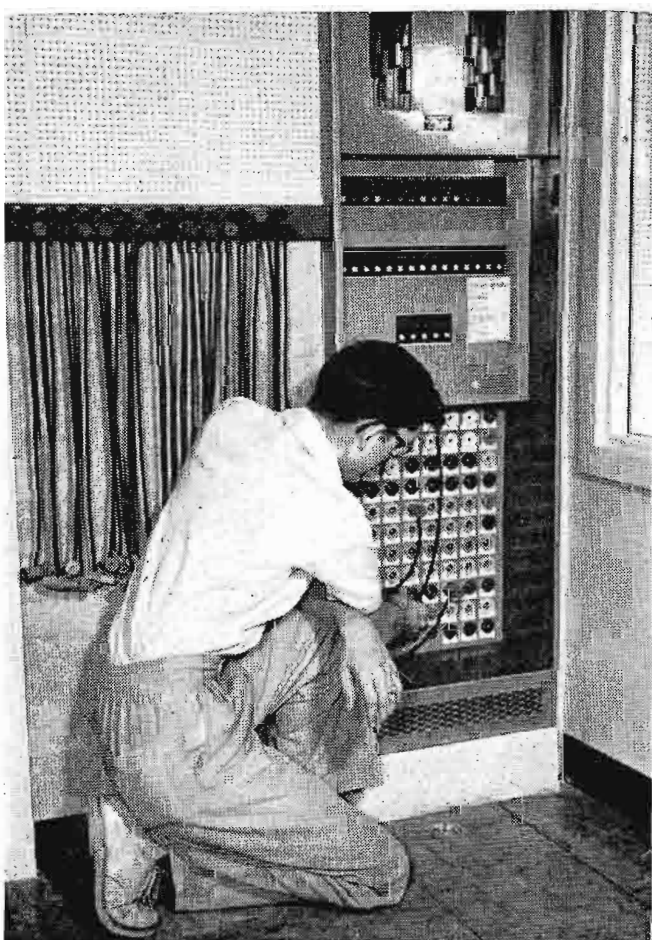
FIG. 14. Davis Dimmer and Switchboard Panel with rack of Connecting Cords for selecting studio lighting combinations.
