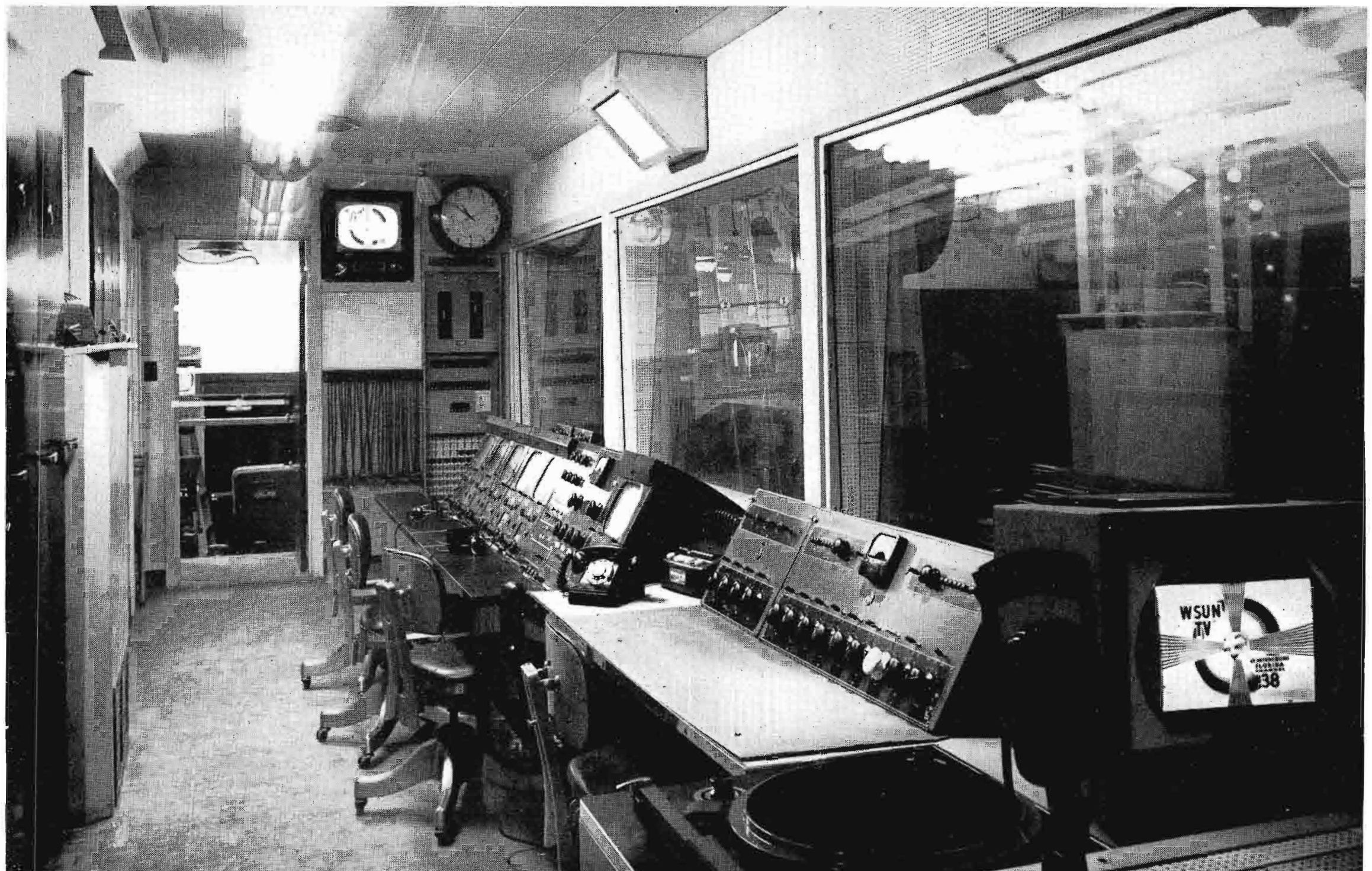
FIG. 12. Studio Control Room. From far end, console equipment consists of two monitors for studio cameras, two film camera monitors with control units, a line monitor with TS-10A switcher, two console housings comprising the TC-4A switchers and a preview monitor. Moving forward from the telephone and intercom unit is the BCM-1A audio mixer and the BC-2B audio consolette. An RCA utility monitor and 70-D transcription turntable are in the foreground. To the left is studio rack equipment and the director's box. In the background is the film room and the studio lighting control panel.
